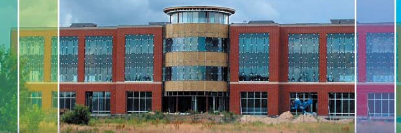
Opening this September, the Ontario AgriCentre™ is being designed specifically to help farm organizations be more effective and efficient through the sharing of facilities and resources. A special feature of the building will be a modern Media Centre that can be used for media events and live broadcasts from the building.
